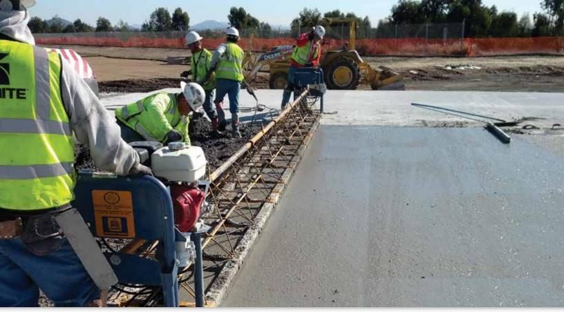
The use of forms did not prevent Granite from using their slipform crews and equipment. A G & Z slipform paver was first used to place the high temperature concrete by straddling the forms and placing separate pavements that were either 30' or 34' apart. Once the original slabs were set and cured, the slipformer traveled on the existing pavements to place and finish the 30' and 34' gap sections.
