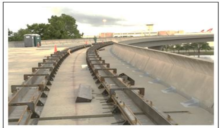
Shorter forms (5ft lengths) were used for radius pours
