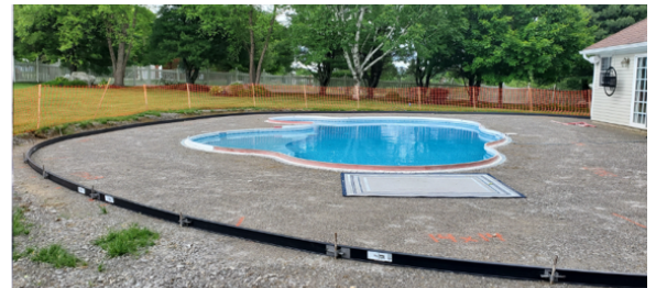
Pool Deck Forming- Using Poly Meta Forms®
