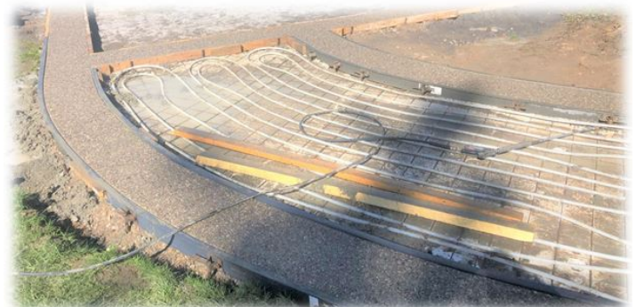
Poly Meta Forms® used to form exposed concrete border.
