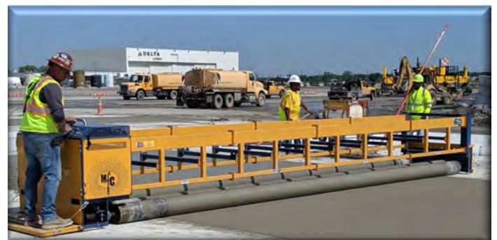
When concrete paving project requires a power screed, MFC now offers a choice between a truss machine and a roller tube model.
