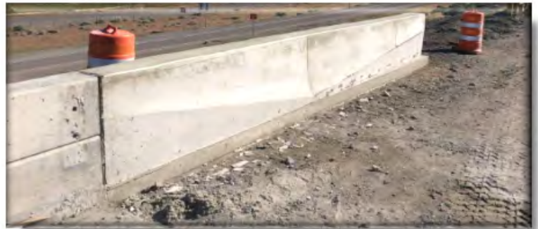
"NDOT I-80 Repave and Safety Upgrade"
